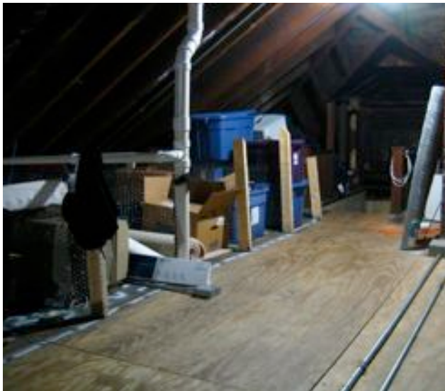
Days of hard work on the parts of Lyall Wallerstedt, John Perleberg, and Emman Mascarinas payed off with the new creation of storage spaces for brothers living in the house.
